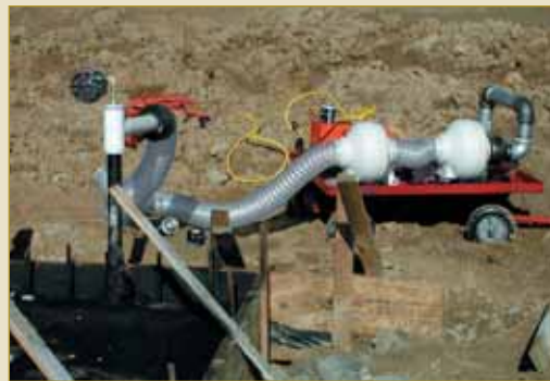
1. Equipment set-up for smoke test
