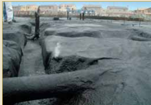
3. Puncture detected by smoke
