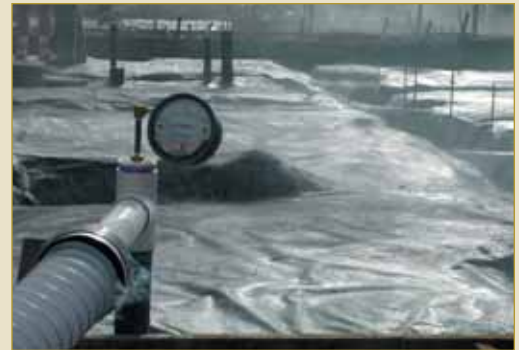
2. Starting smoke test procedure
